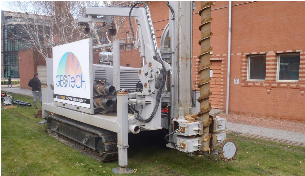
Figure 1: Prototype drill rig on Leicester demo site
